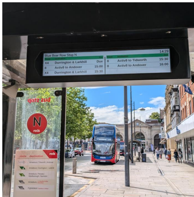
A PATWIS display driven by r2p Systems back office in Salisbury
